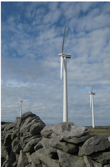
Inis Meáin Co-Op wind farm installed 2002
